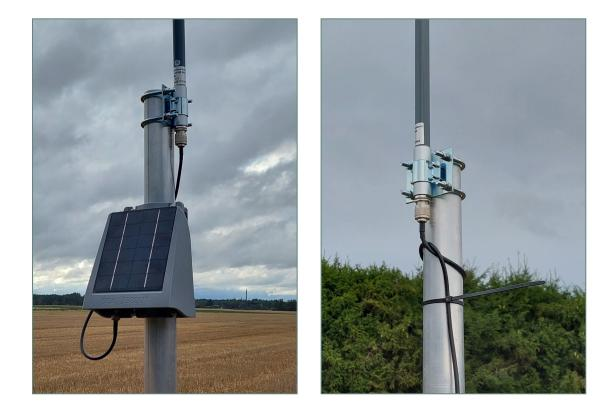
If you're using a short antenna cable, slip the Receiver onto the pole and tighten the backplate screws just a little. Add the Antenna to the pole. An omnidirectional antenna must sit on the highest end of it, having the highest u-bolt just 1 cm (½ inch) below the top - otherwise the pole itself will interfere with the antenna and cause poor performance. Directive Antennas can be mounted at any point of a pole, but preferably as high as possible.
